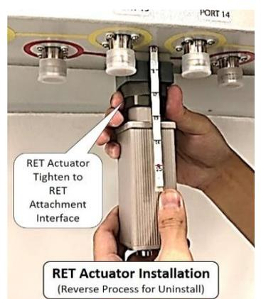
Step 7: Screw and tighten RET cable
