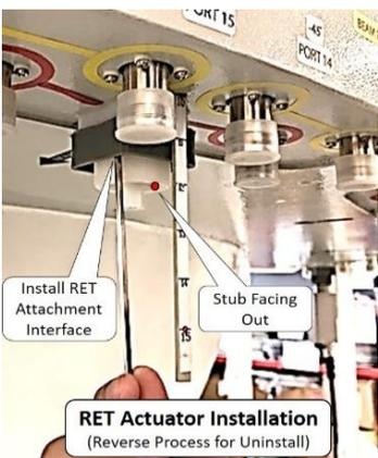
Step 5: RET Actuator stub gap facing out
