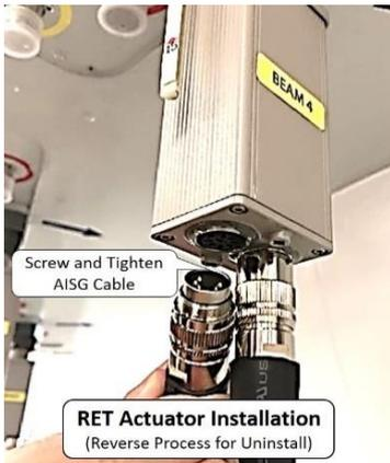
Step 8: RET Actuator installation complete.
