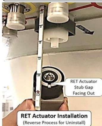
Step 6: RET Tighten to attachment interface
