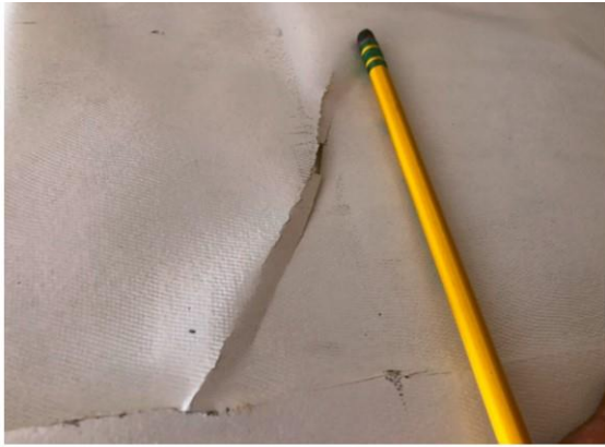
Fibrous Glass Fabric layer Damage Only
