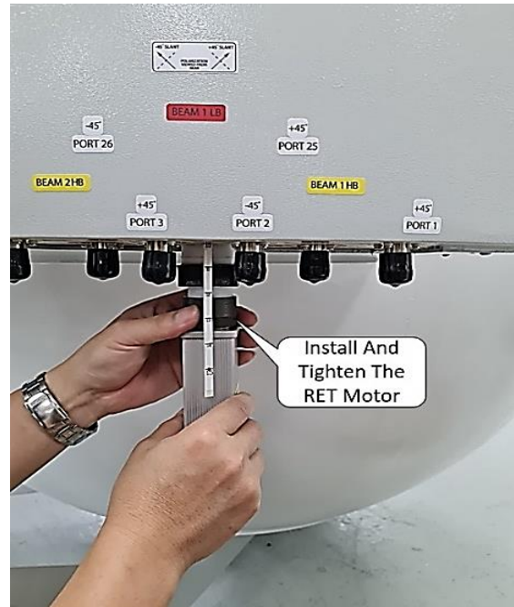
Step 4: Install And Tighten The S-RET Motor
